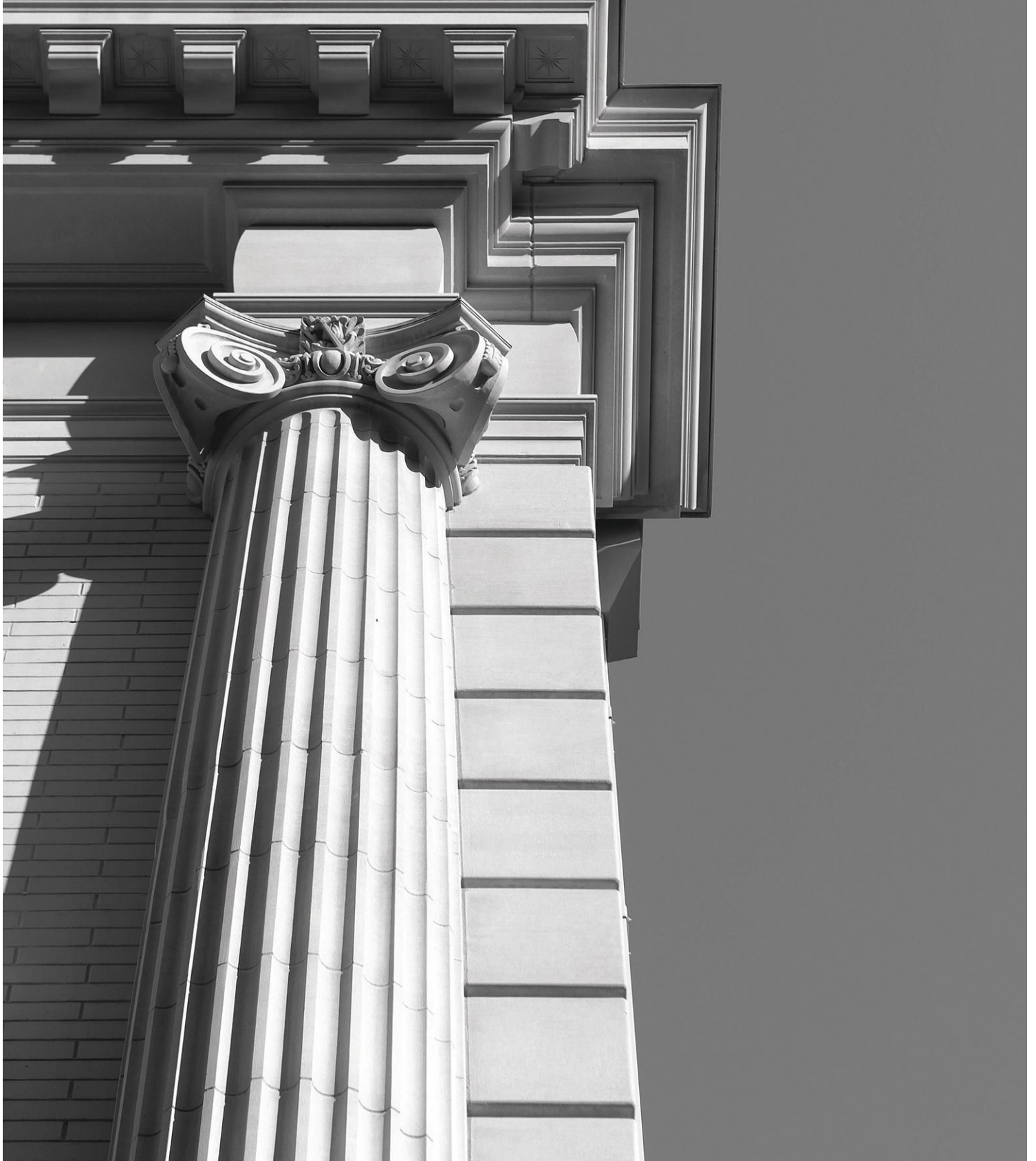
A planer was used to plane the circular shape of the column and the flutes.
